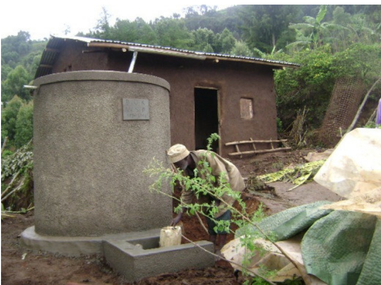
Photos: Kaburabuza at his house before renovation and after renovation with the tank constructed by KDWSP
